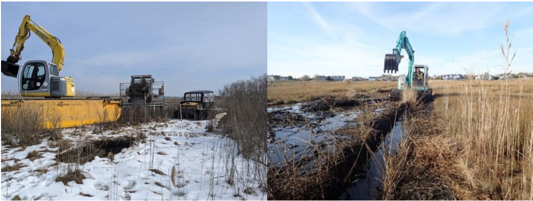
Left: Excavator creating a micro-pool and placing the sediment for transport. Right: Cleaning a tidal creek.
