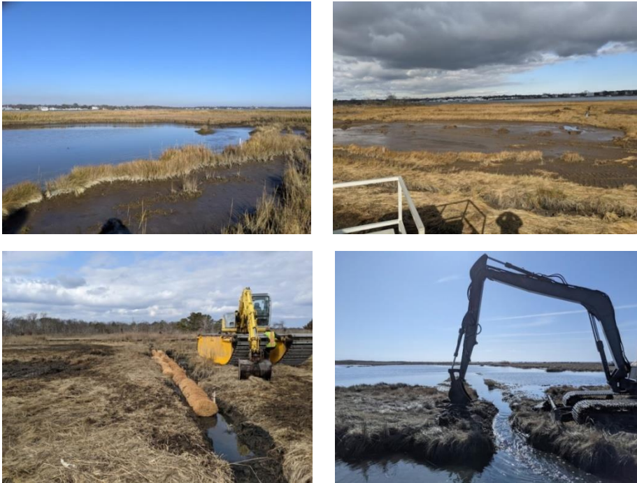
Top-Left; A large panne prior to drainage channel and runnels, Top-Right; Surface after drainage channel and runnels installed. Bottom-Left; Filling of ditches with coir logs. Bottom-right: Immediate aftermath of a runnel being created.
