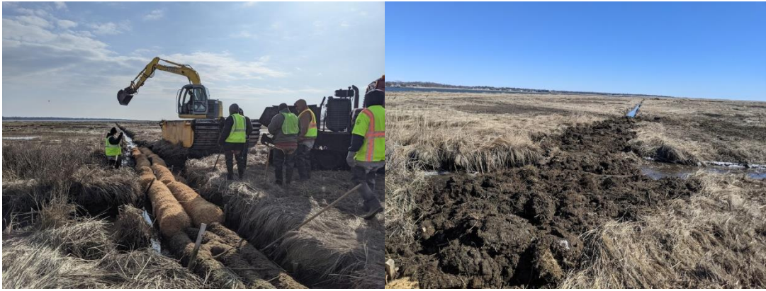
Left: Coir logs placed inside a pre-existing ditch. Right: Marsh material placed on top of coir logs to fill a ditch.
